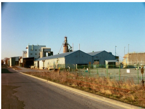
Former Paper Mill - Downtown City of Thorold, Niagara Region
